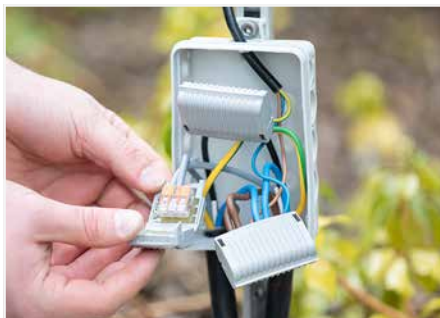
Connecting a bollard light
