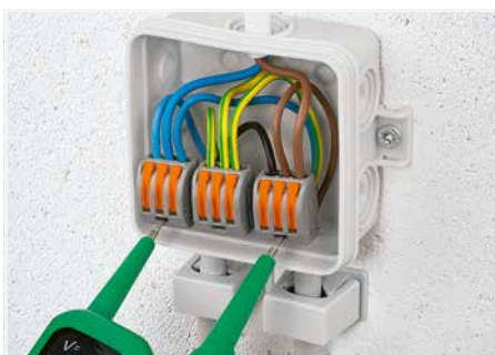
Testing the wired connectors.
