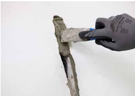
Close the damaged area discreetly.
